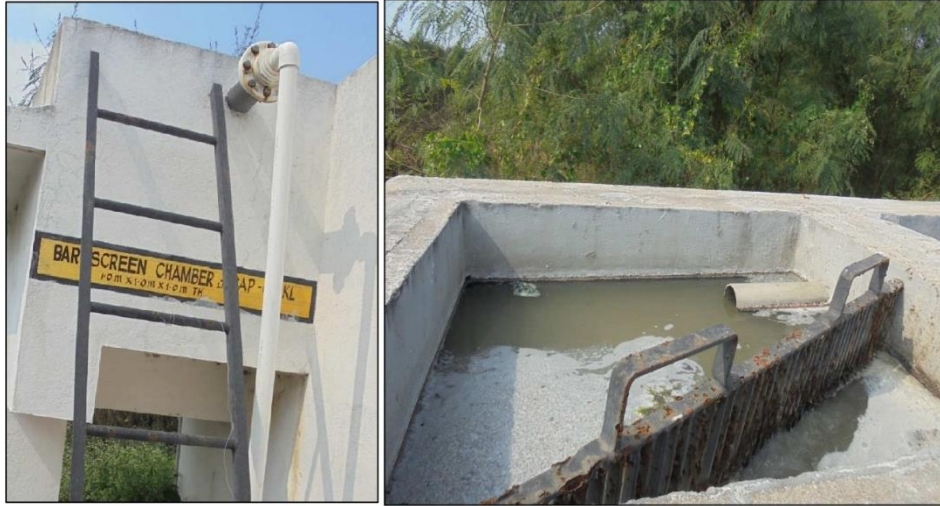
Bar Screen Chamber at STP
