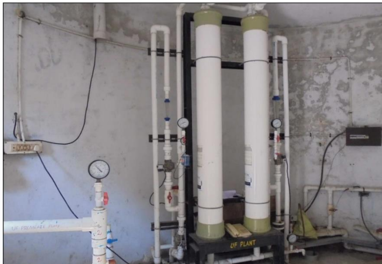
Aeration Tank at STP
