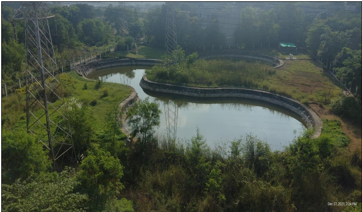
Rain Water Harvesting Pond within the Campus
