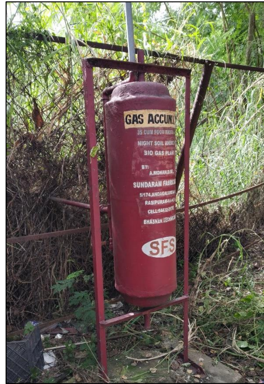
Food Waste Crusher at Bio Gas Plant Gas Accumulator at Bio Gas Plant
