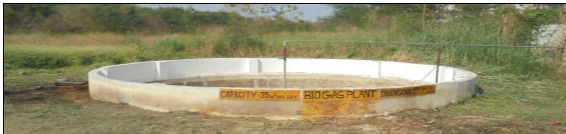
Bio Gas Plant (35 Cu. M Capacity) within the campus
