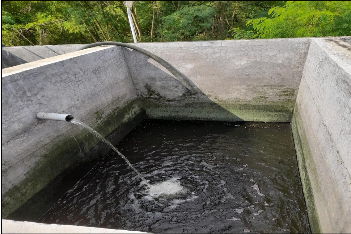
Clarified Water Storage Tank
