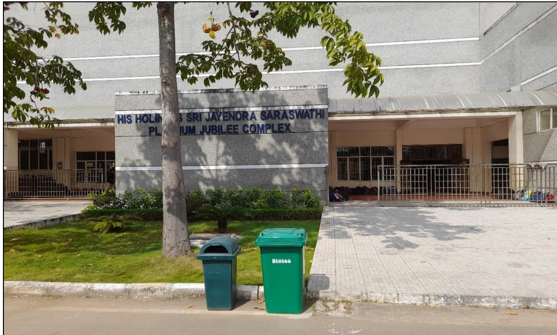
Waste Segregation System
