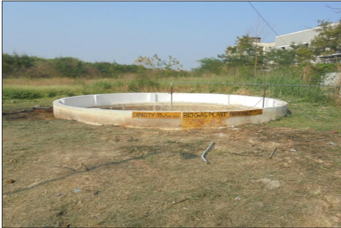
Bio Gas Plant
