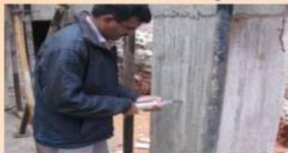
REBOUND HAMMER TEST
