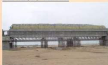
LOAD TEST ON PSC DECK OF RAILWAY BRIDGE
