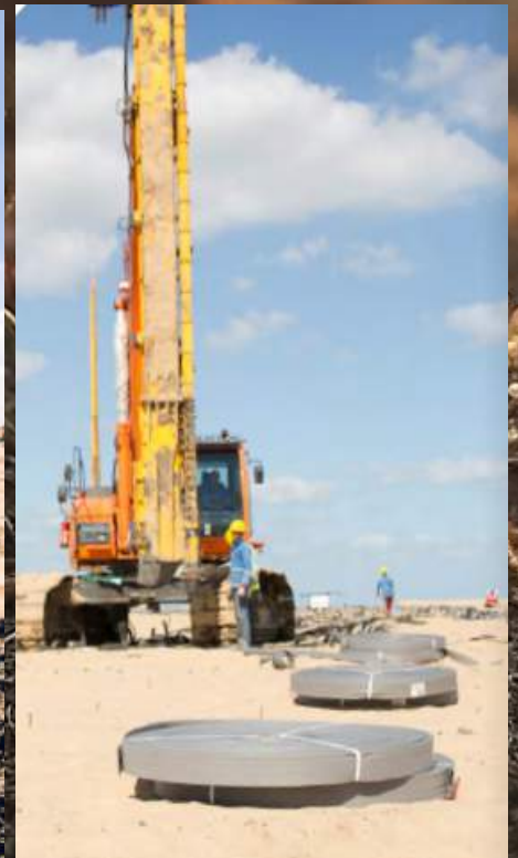
INSTALLATION PROCESS OF PVD AT SITE
