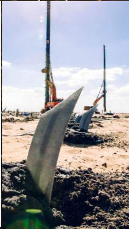
INSTALLATION PROCESS OF PVD AT SITE
