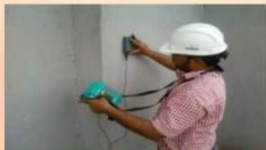
SCANNING OF REBARS
