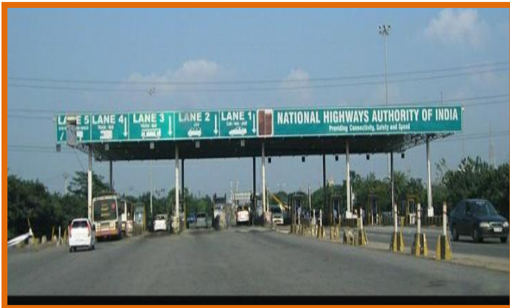
Fig. 2.3 Nemili Toll Plaza near Sriperumbudur
